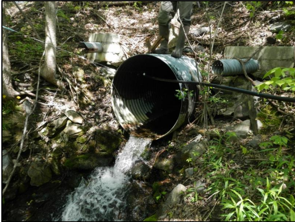
V-FH-S-25 Culvert Outlet
