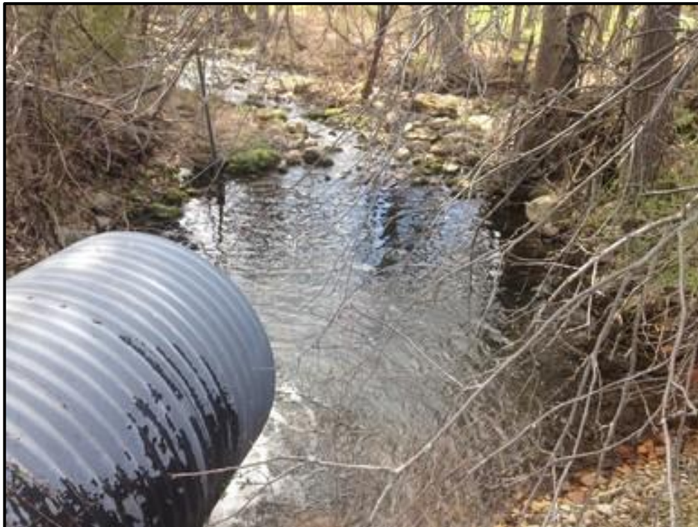
T-CL-S4 Culvert Outlet / Downstream Channel
