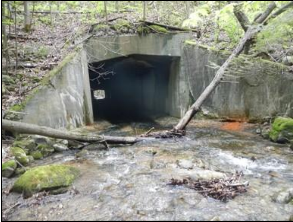
V-SH-S-14 Culvert Inlet
