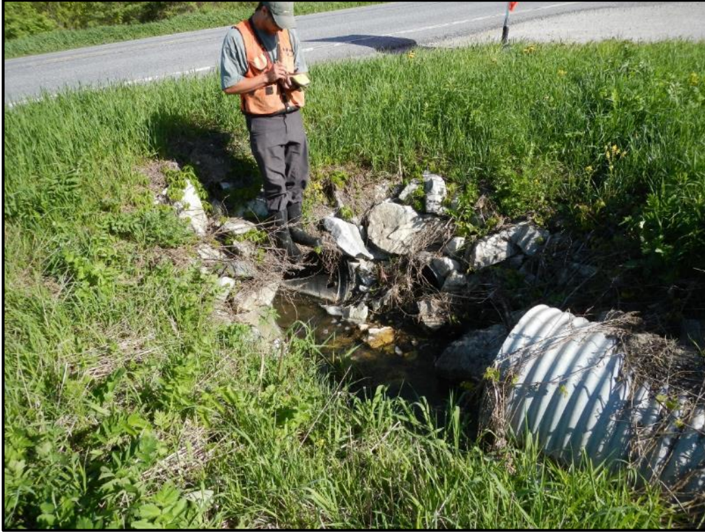
V-WH-S-4 Culvert Inlet
