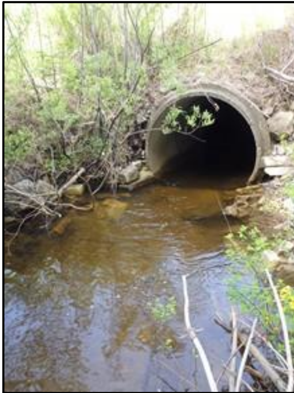
T-MH-AS-20 Culvert Outlet
