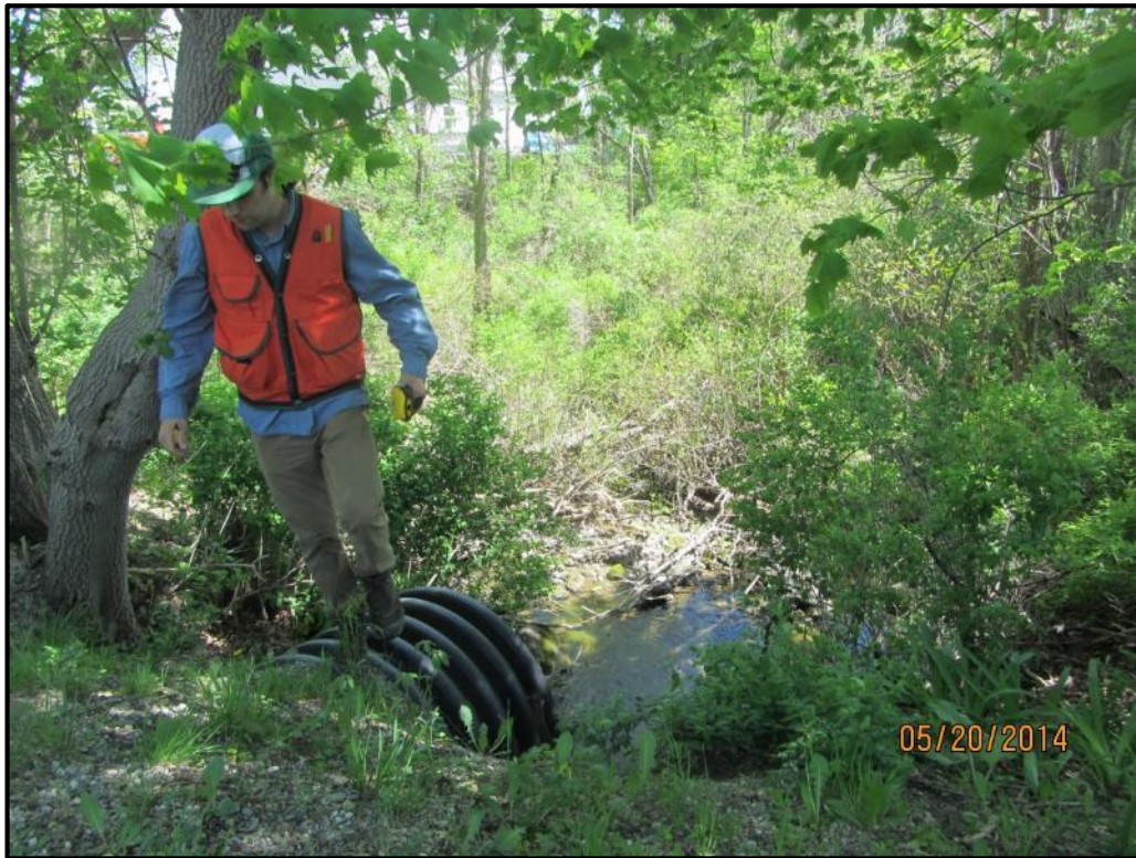
V-BE-AS-10 Culvert Outlet
