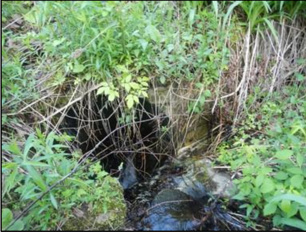
V-SH-S-16 Culvert Inlet
