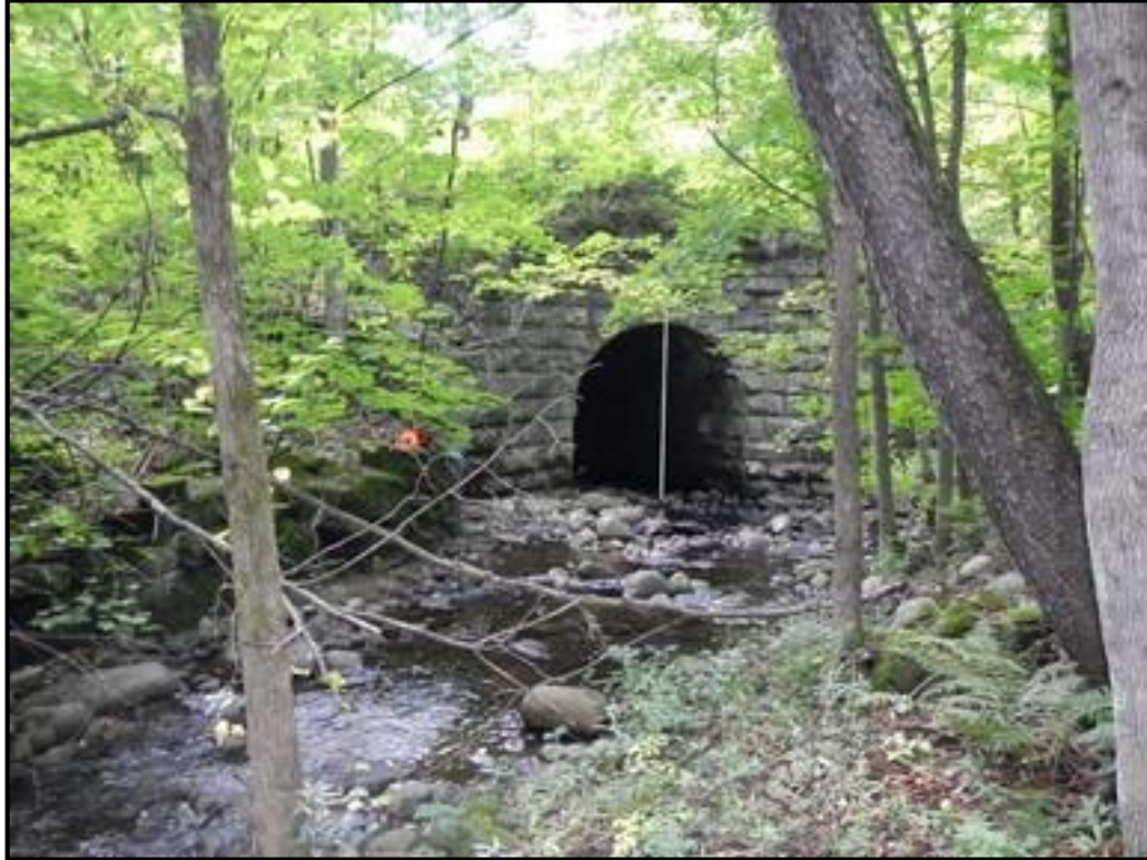
T-SH-S3 Culvert Inlet
