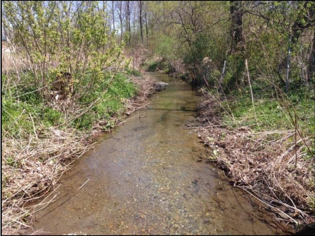
T-WR-S18 Downstream Channel
