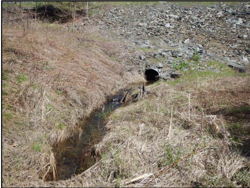
V-FH-S-10 Culvert Outlet
