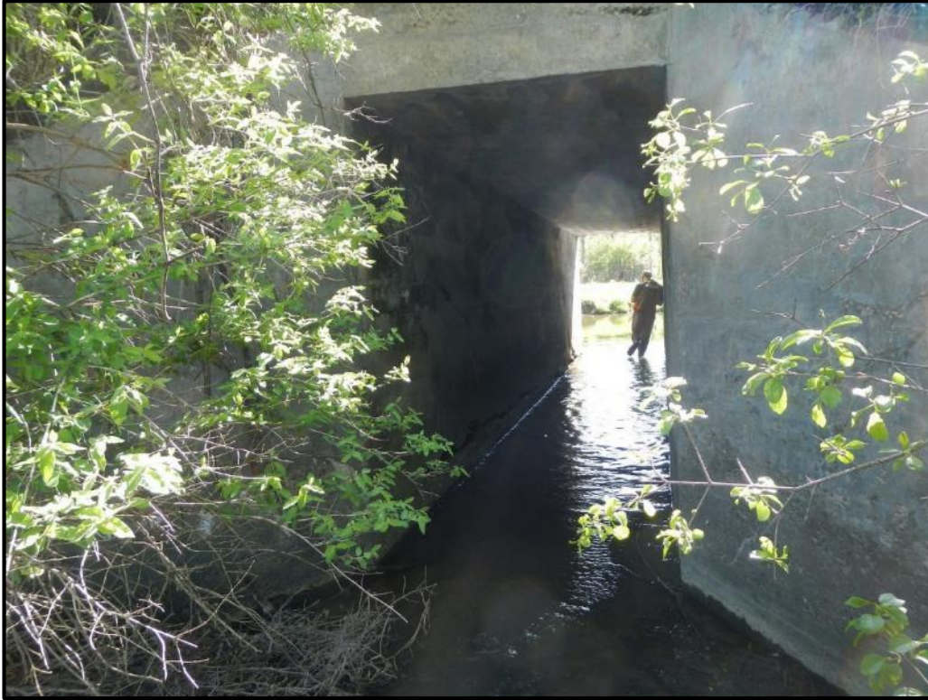
V-BE-S-102 Culvert Inlet
