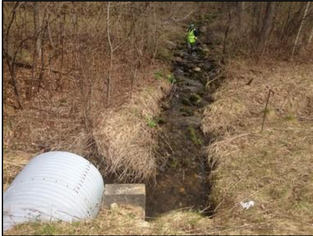
T-CL-S4 Upstream Channel / Culvert Inlet
