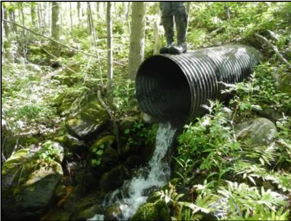
V-SH-S-16 Culvert Outlet
