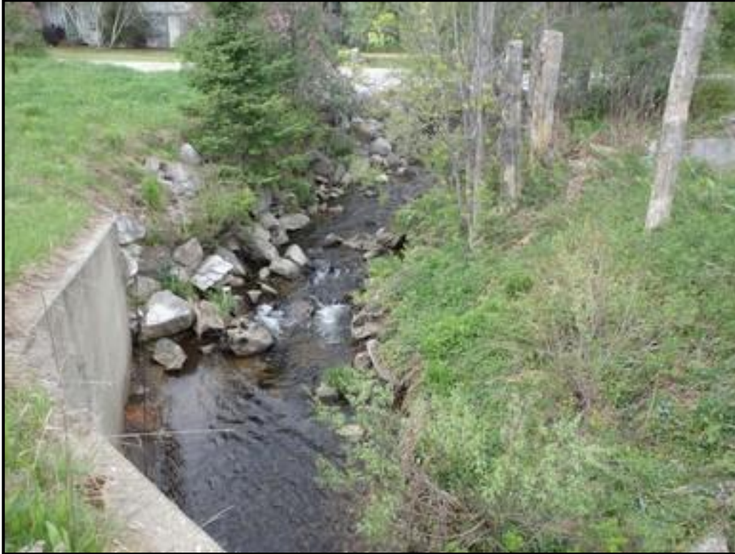
T-MH-S-14 Upstream Channel
