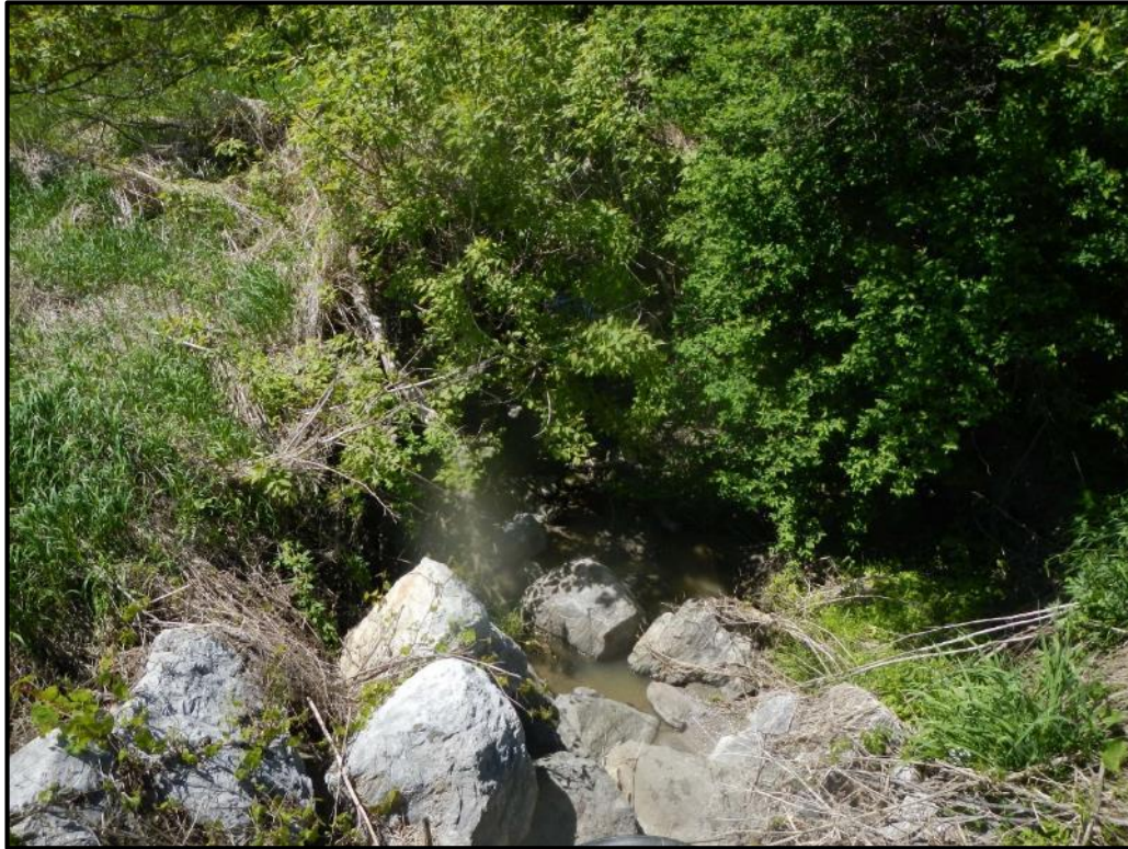
V-BE-S-109 Downstream Channel
