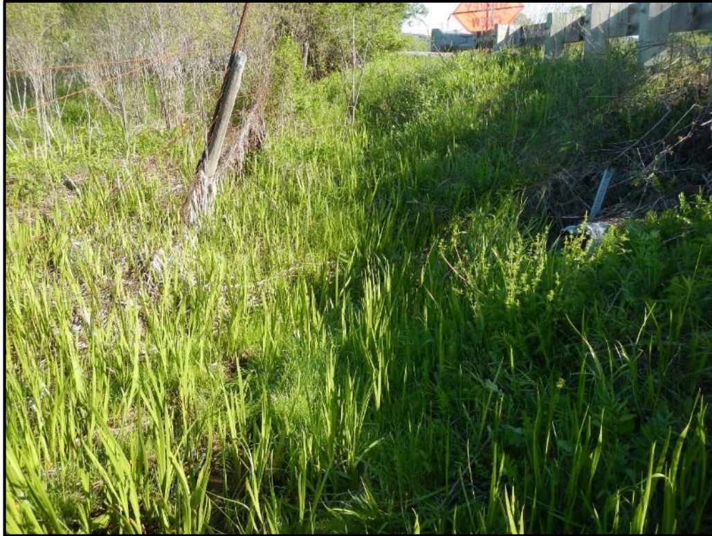
V-BE-S-100 Culvert Inlet / Upstream Wetland V-BE-AW-100
