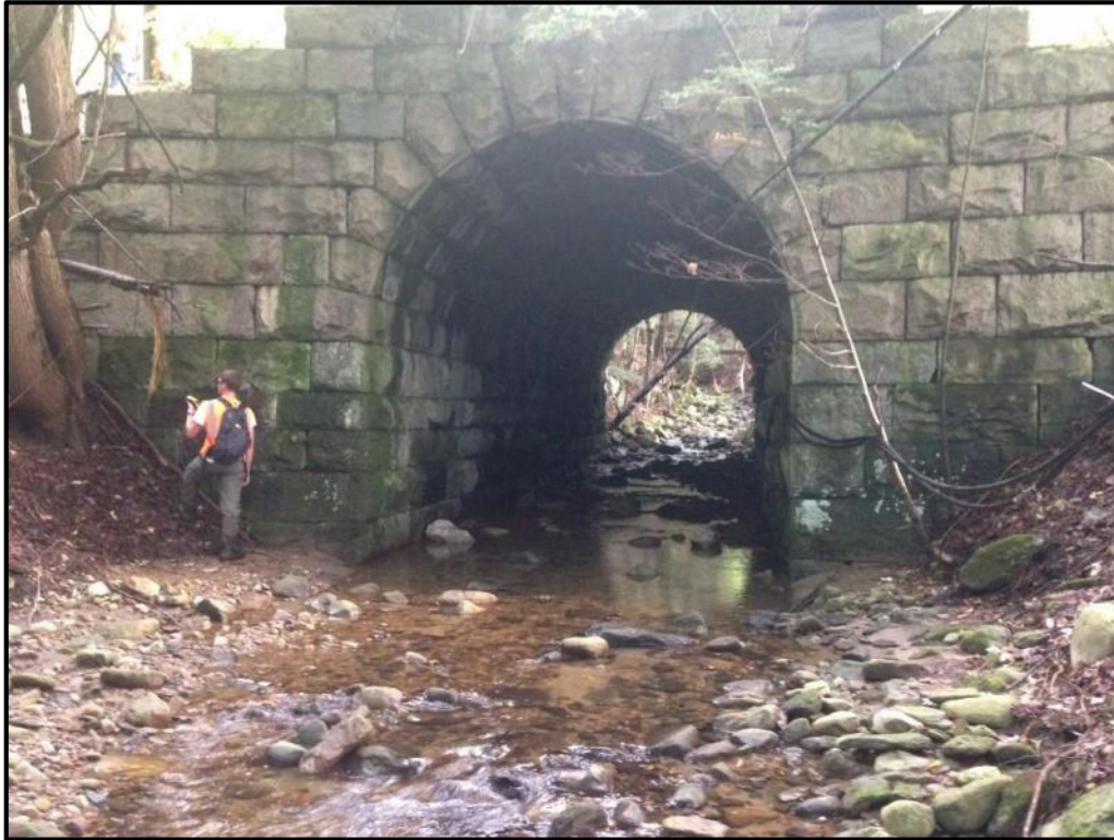
T-SH-S2 Upstream Channel and Arc Culvert
