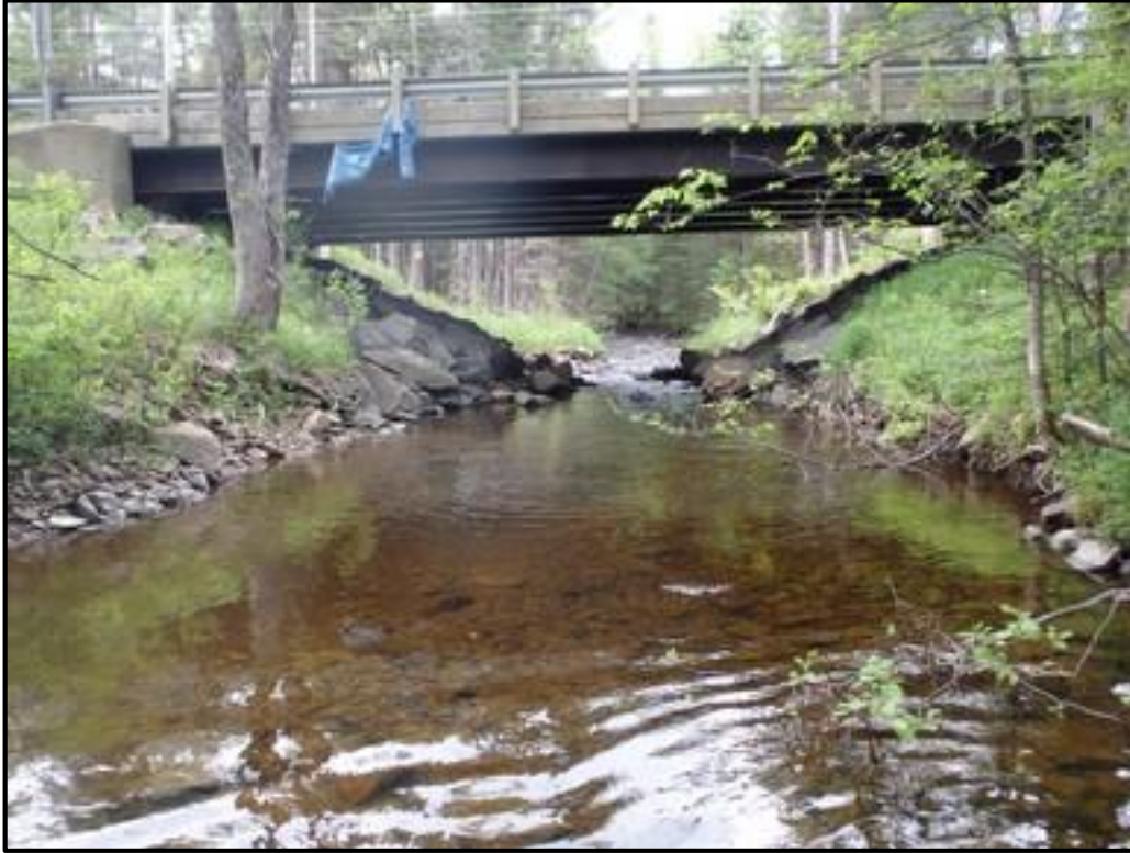
T-MH-S28 Downstream Channel
