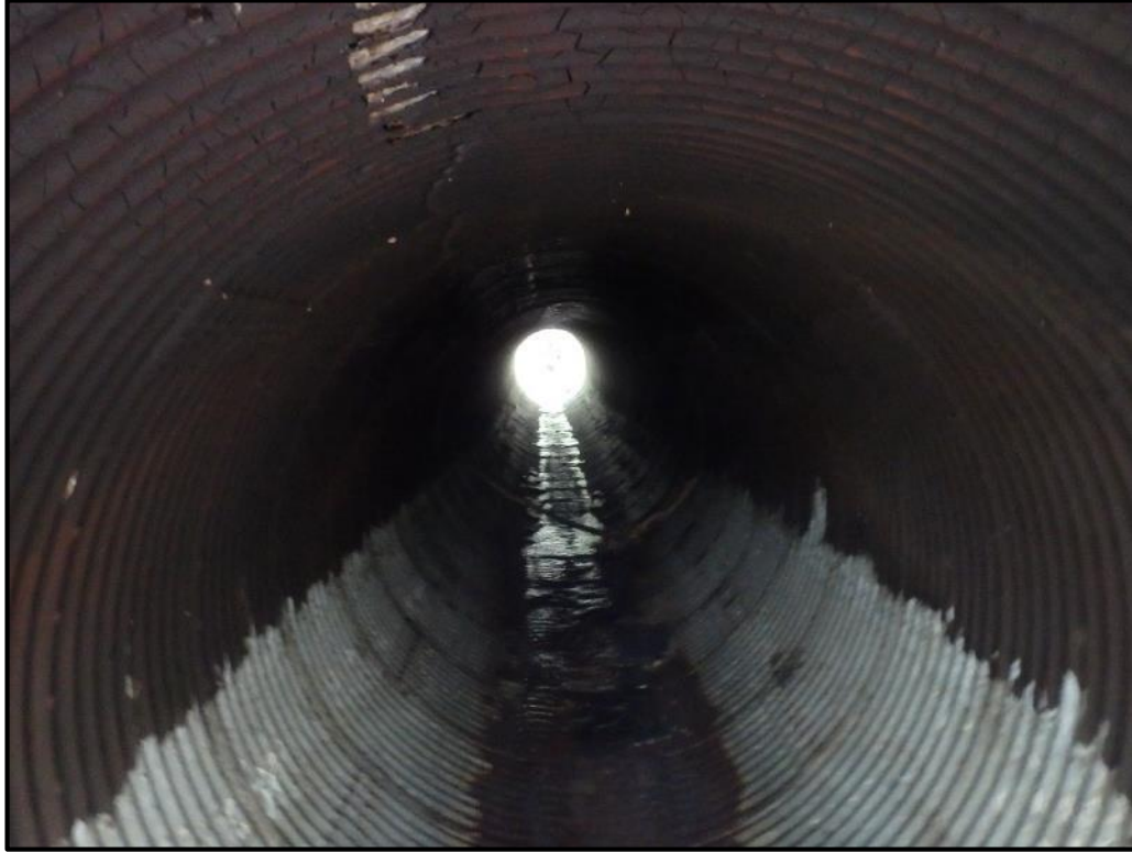
T-MH-S1 Culvert Interior
