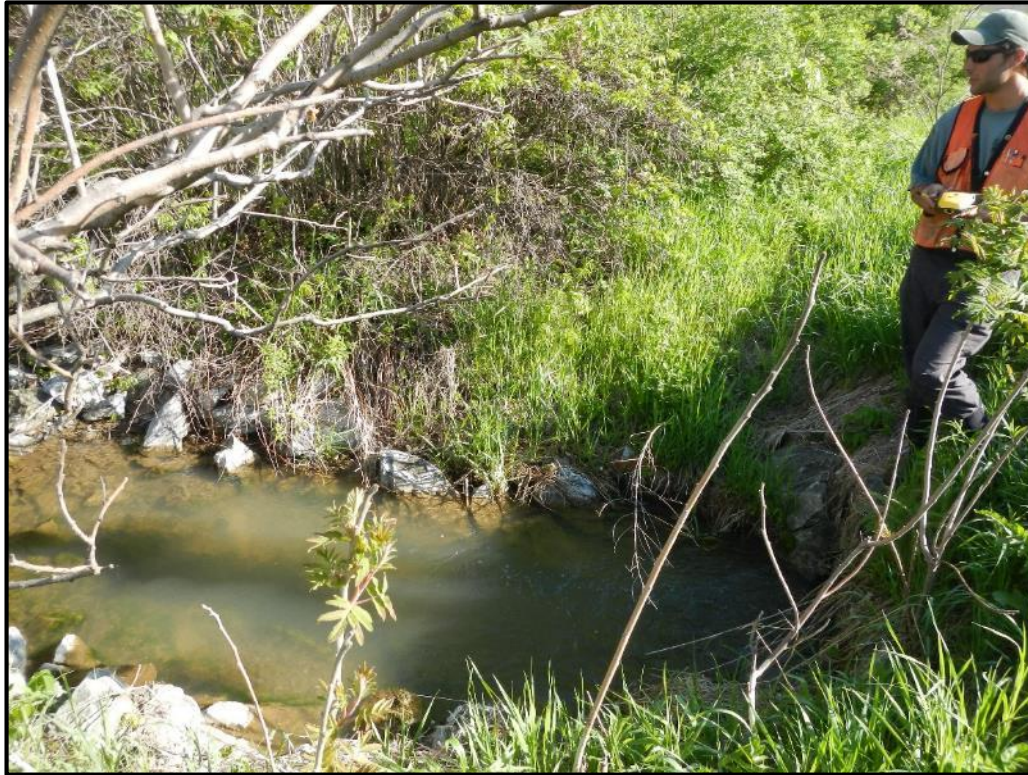
V-WH-S-4 Culvert Outlet
