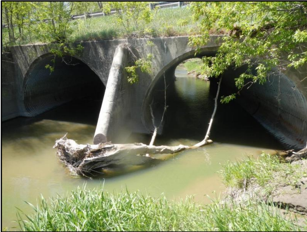
V-BE-S-106 double culvert inlet
