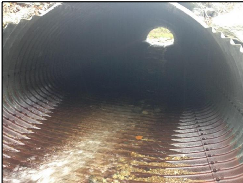
T-LU-S4 Culvert Interior
