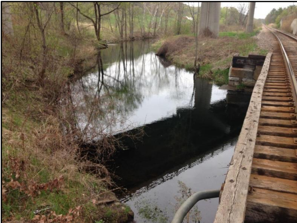
T-WR-S29 Upstream Channel
