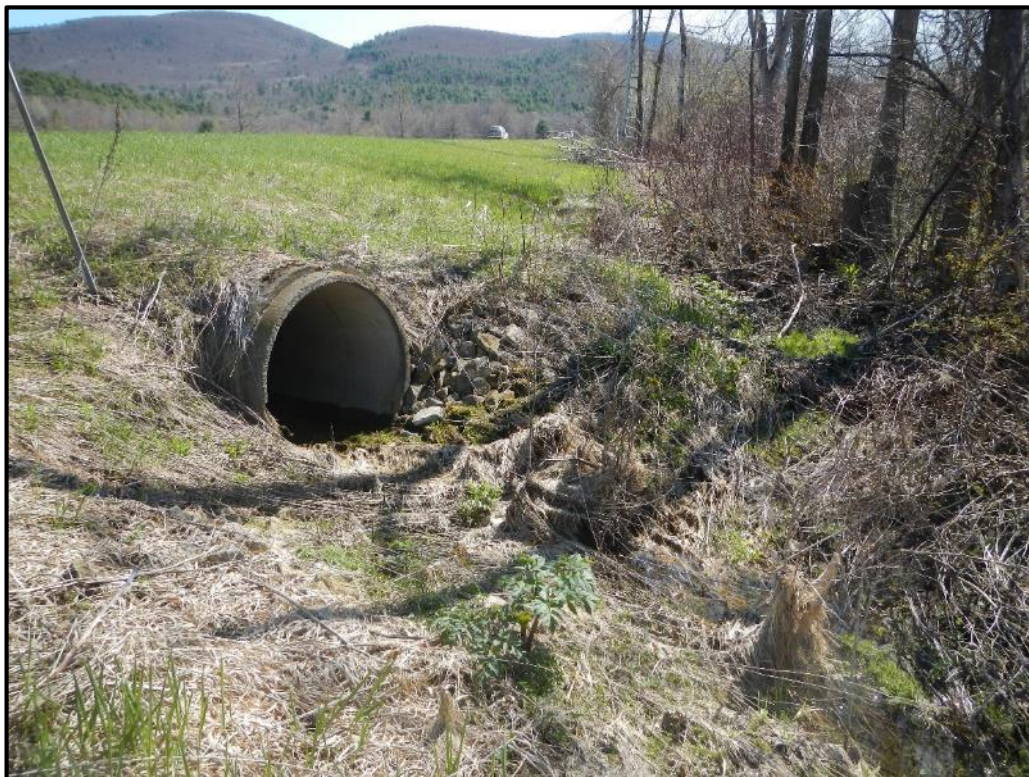
V-CN-S-4 Culvert Outlet
