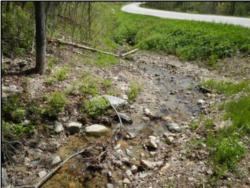
V-WA-S106 Culvert Inlet
