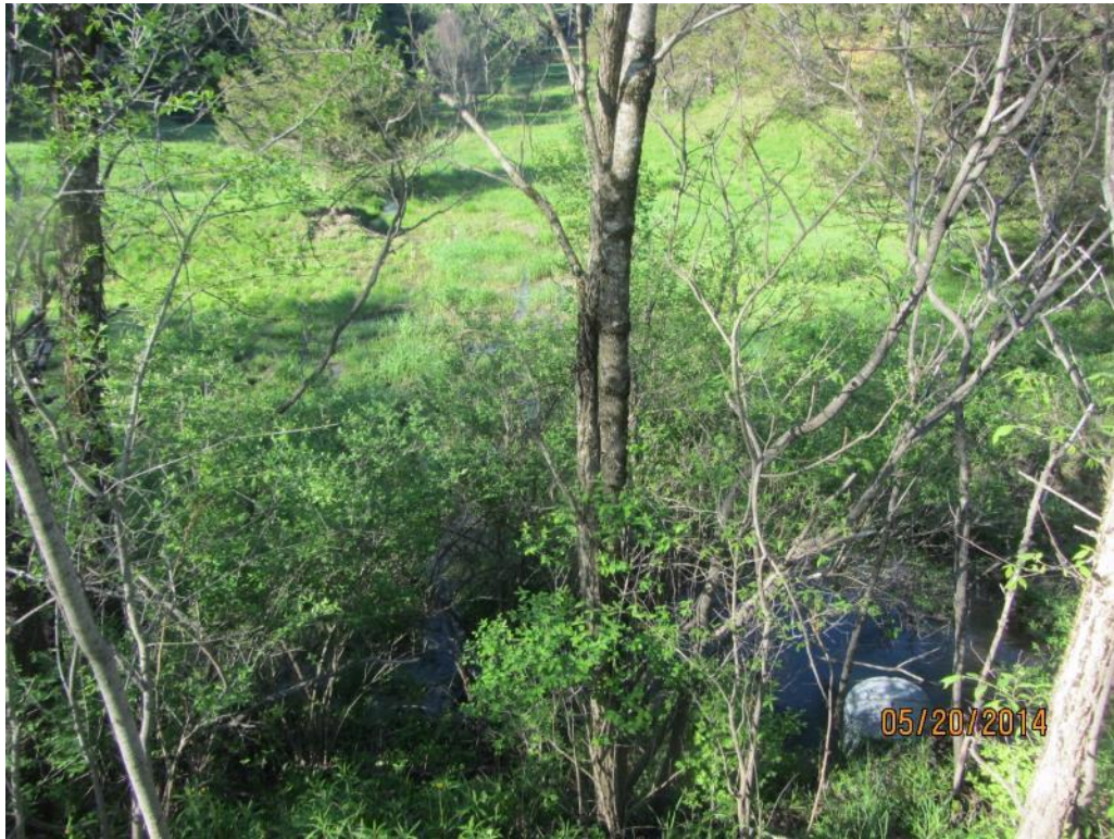
V-BE-AS-3 Culvert Outlet / Downstream Wetland (V-BE-AW-4)
