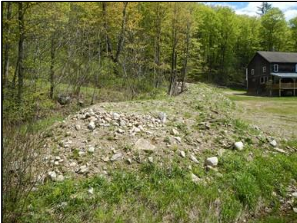
V-WA-S105 Upstream Flood Berm
