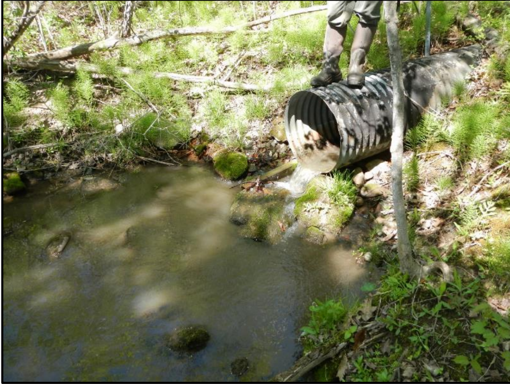
V-WH-S-2 Culvert Outlet
