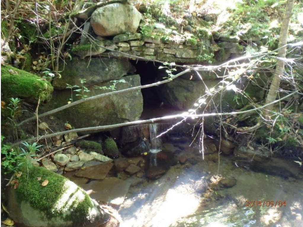
T-SH-S7 Culvert Outlet
