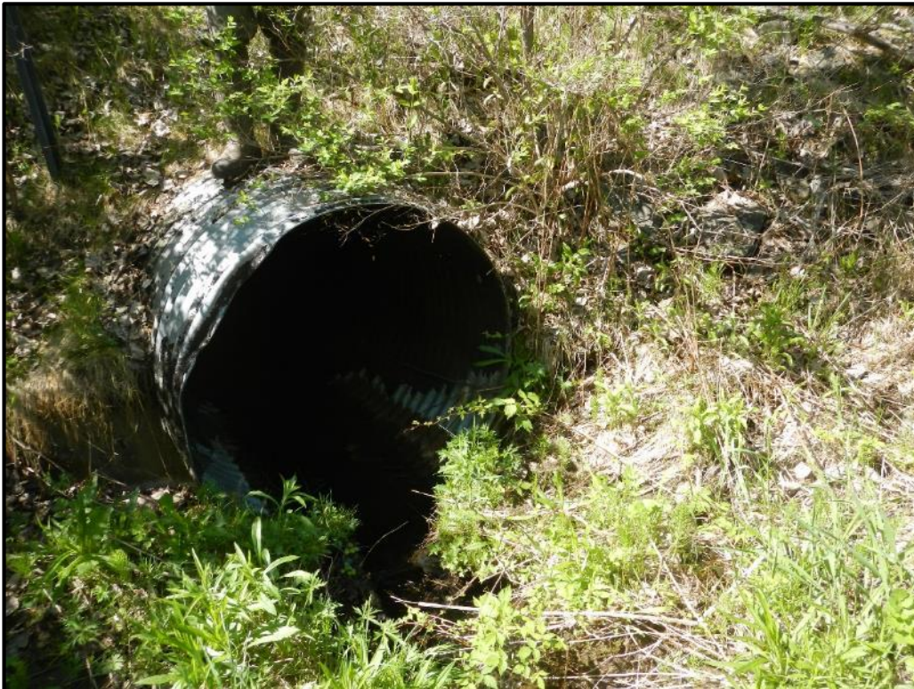
V-FH-S-17 Culvert Inlet
