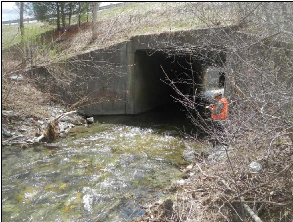
V-CN-S-8 Box Culvert
