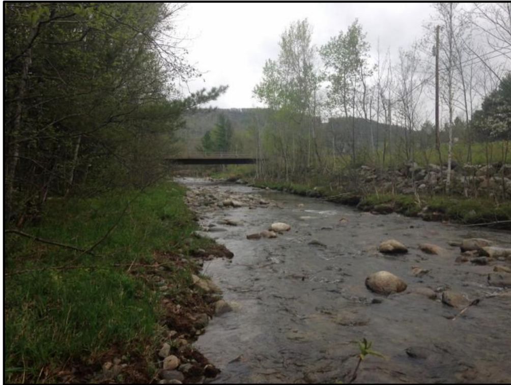
T-LU-S2, View toward VT Route 100 Bridge
