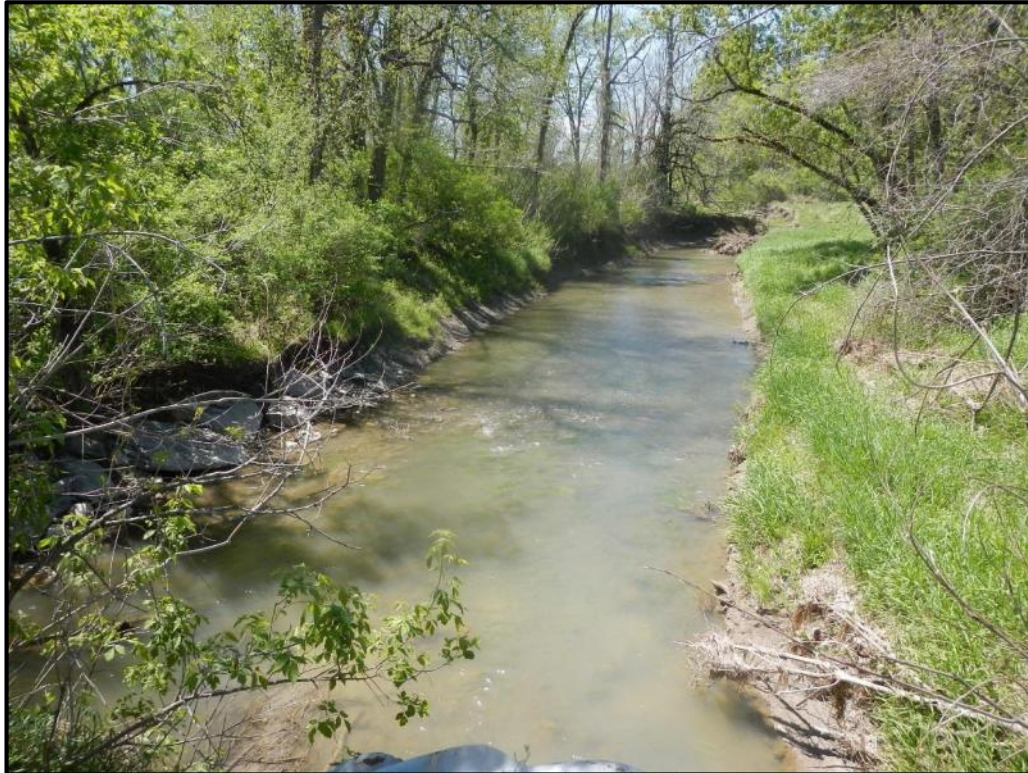
V-BE-S-106 Downstream Channel
