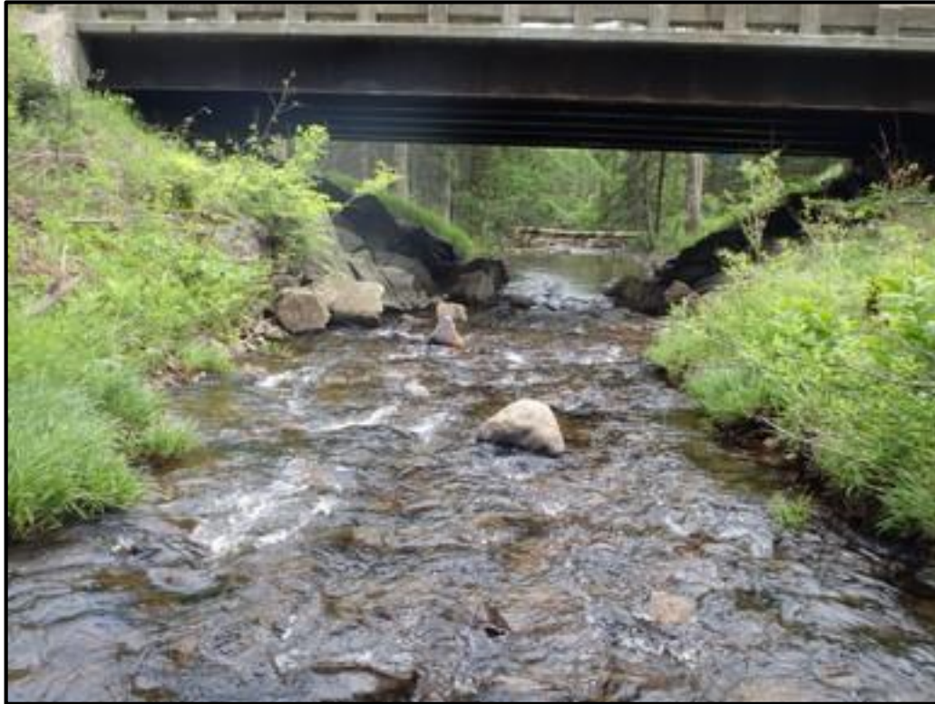
T-MH-S28 Upstream Channel
