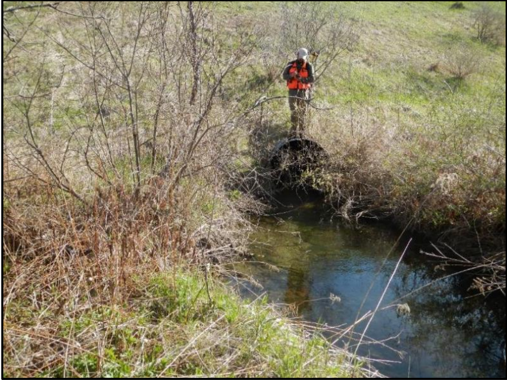
V-CN-S-12 Culvert Outlet
