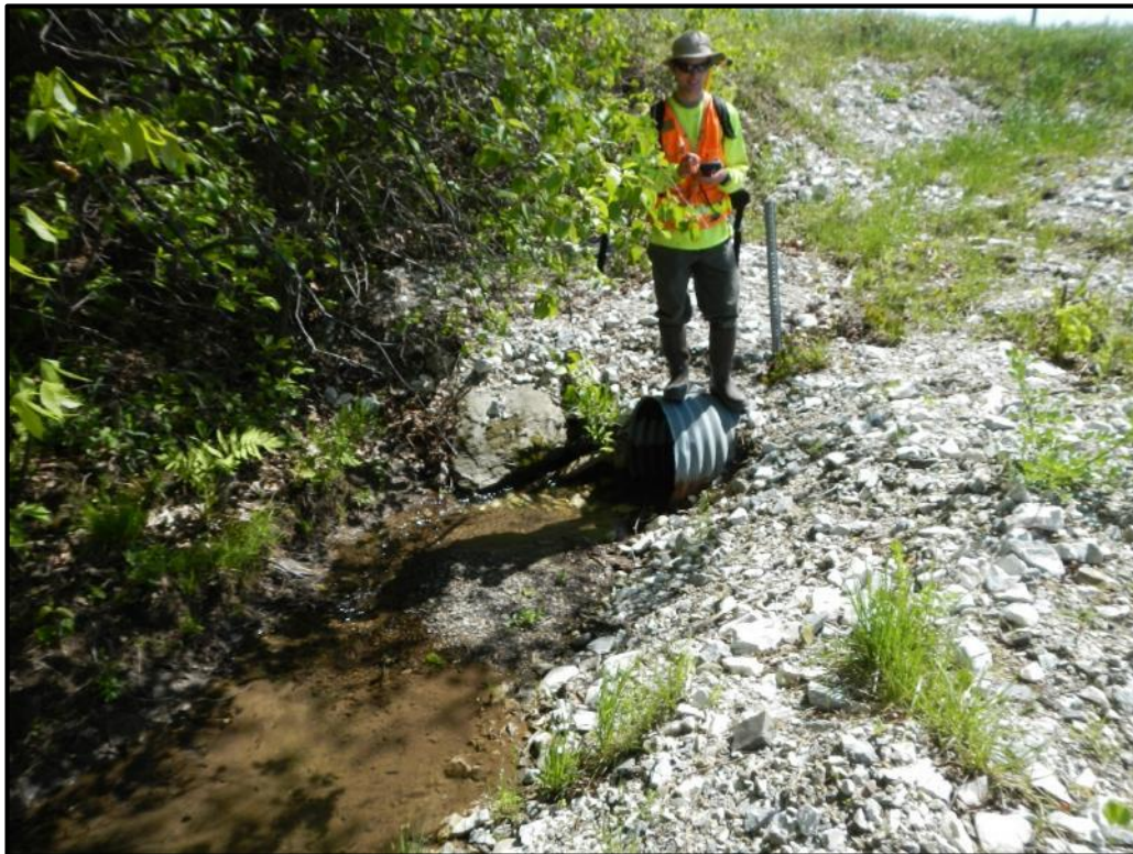
V-WH-S-2 Culvert Inlet
