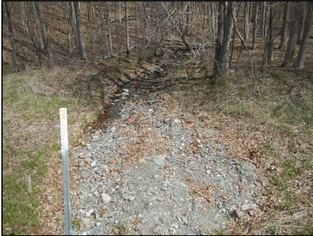
V-CN-S-4 Culvert Inlet
