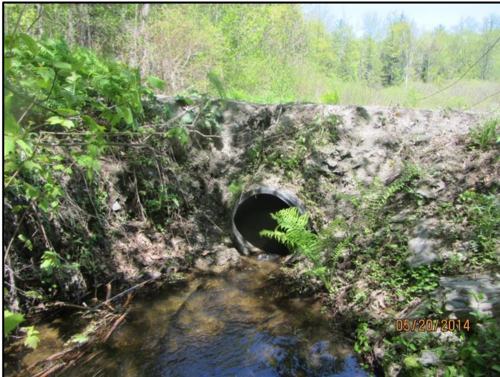
V-BE-S-8 Culvert Outlet
