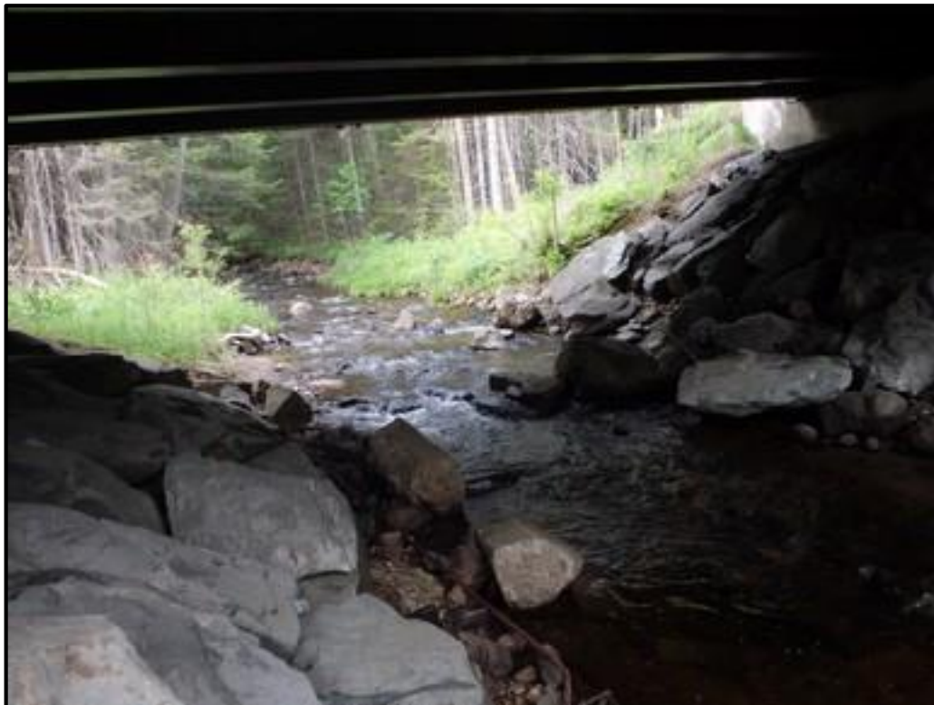
T-MH-S28 Upstream Channel from beneath bridge
