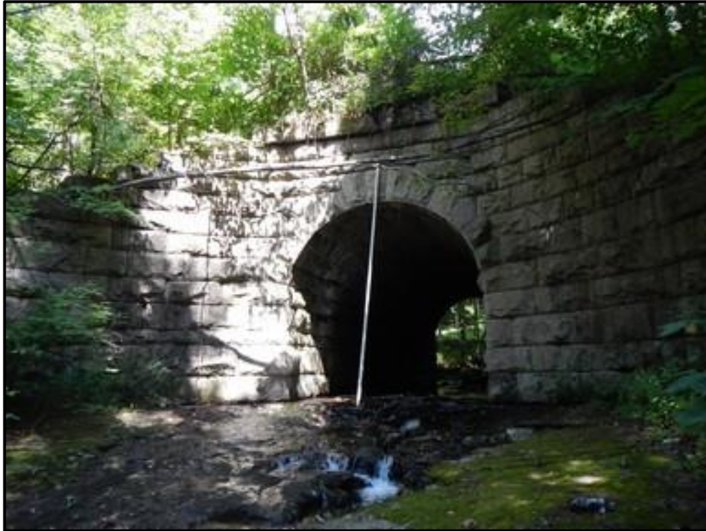
T-SH-S3 Culvert Outlet
