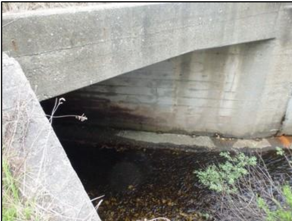
T-MH-S-14 Culvert Inlet
