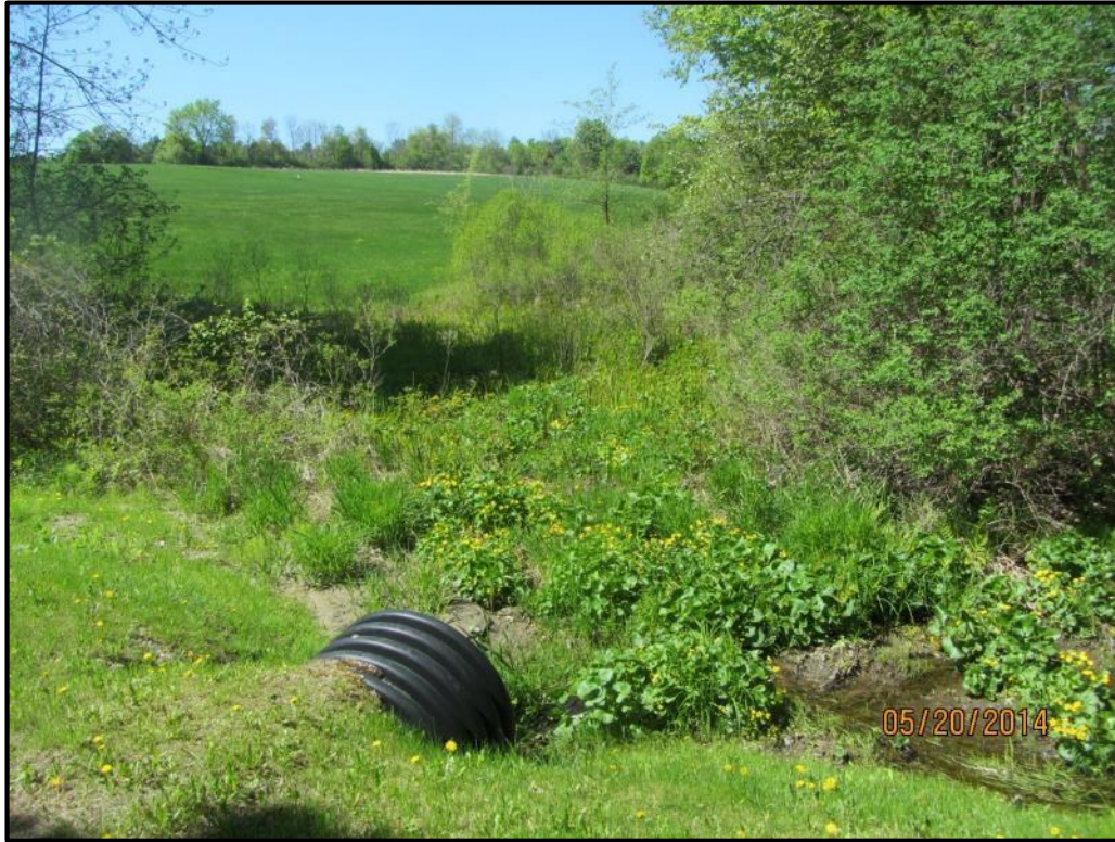
V-BE-AS-10 Culvert Inlet / Upstream Wetland (V-BE-AW-17)
