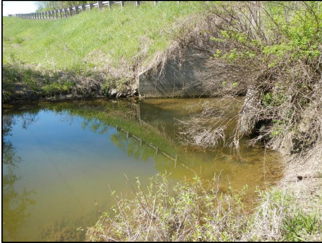
V-BE-S-102 Culvert Outlet
